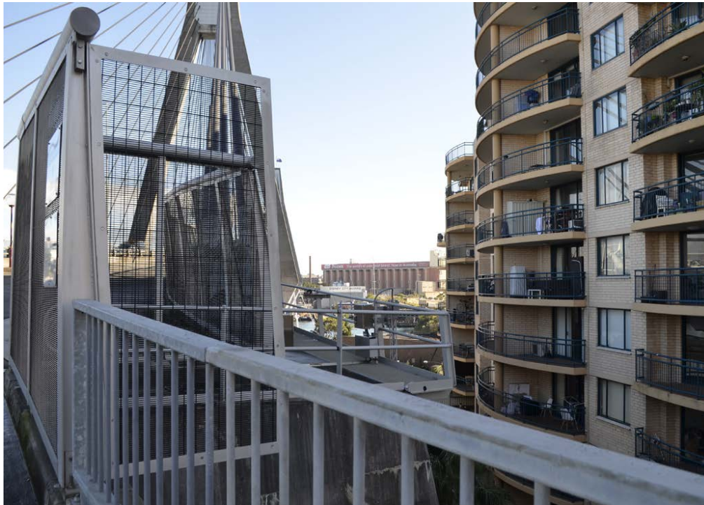
View 30: From Anzac Bridge near eastern pedestrian/cycle ramp entry/exit. Photography by GroupGSA
